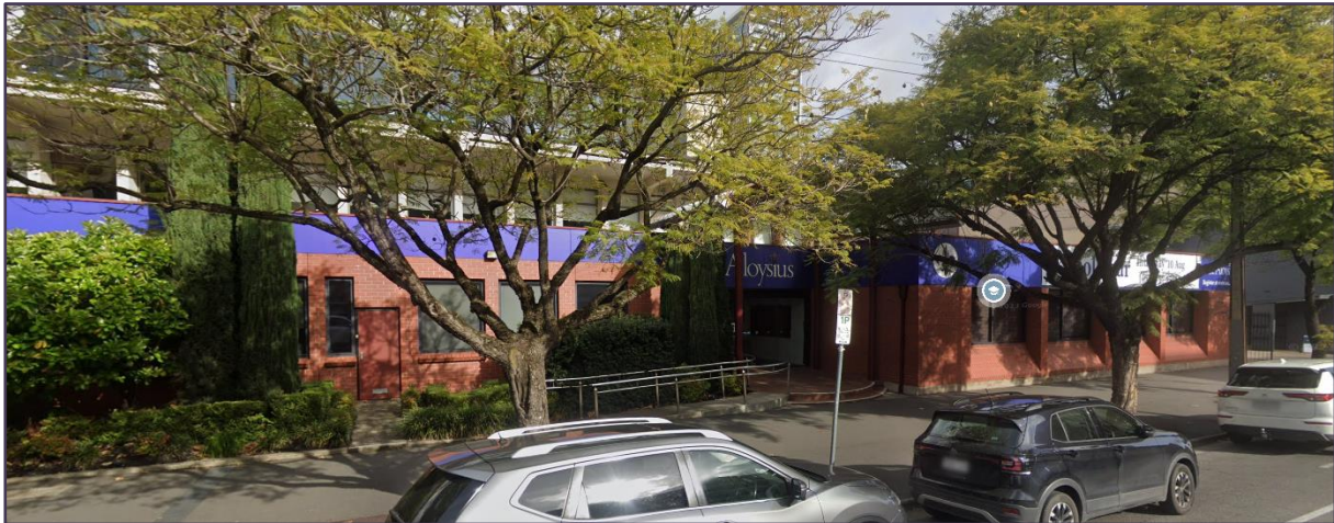
Figure 1 - Subject site view from Wakefield Street
